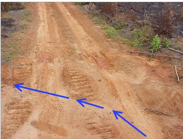
The diverted water is carried off the road and through the wing ditch into a vegetated patch of land which will absorb the runoff.
